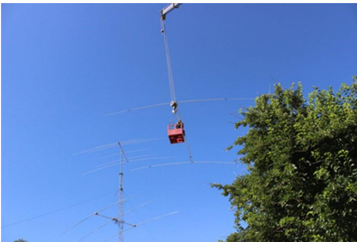
Forty Meter Yagi going up at KE5OG's QTH.
