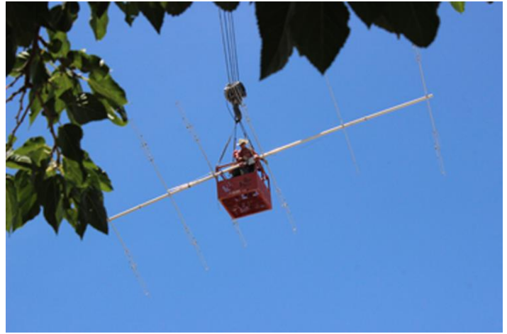
KT-36XA Yagi being lowered at the K5FD (SK) QTH – a monster antenna!
